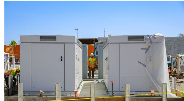
Feb 23, Schneider site work begins
