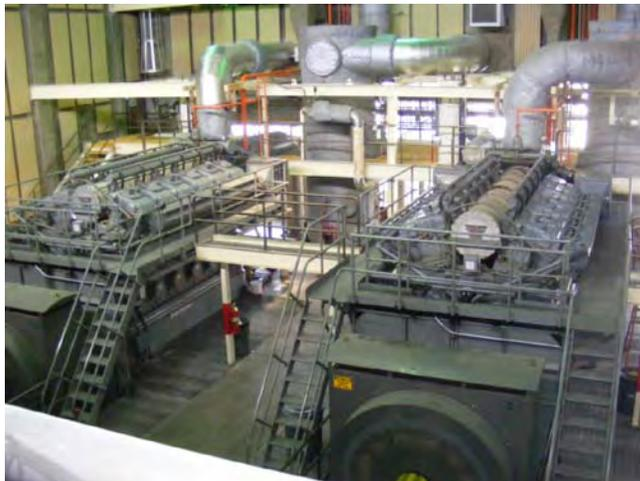
**Figure 9: OCS D Biogas Engines**
