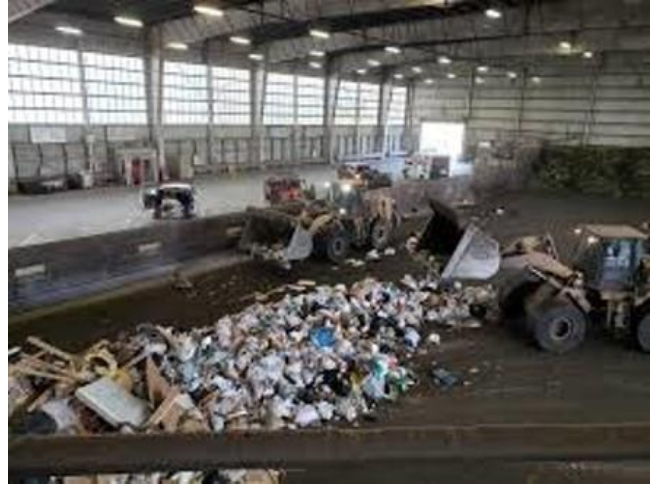
Figure 1: Southeast Resource Recovery Facility (SERRF).
