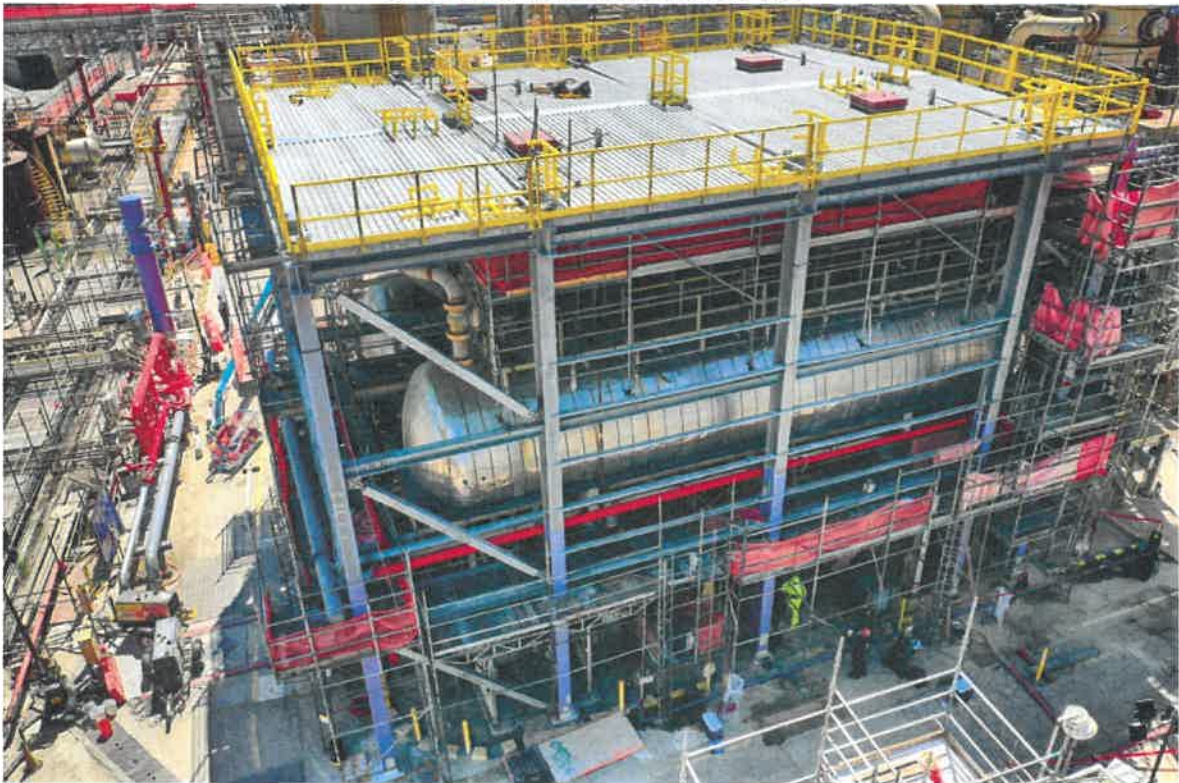
Structure with Roof Panels Set
