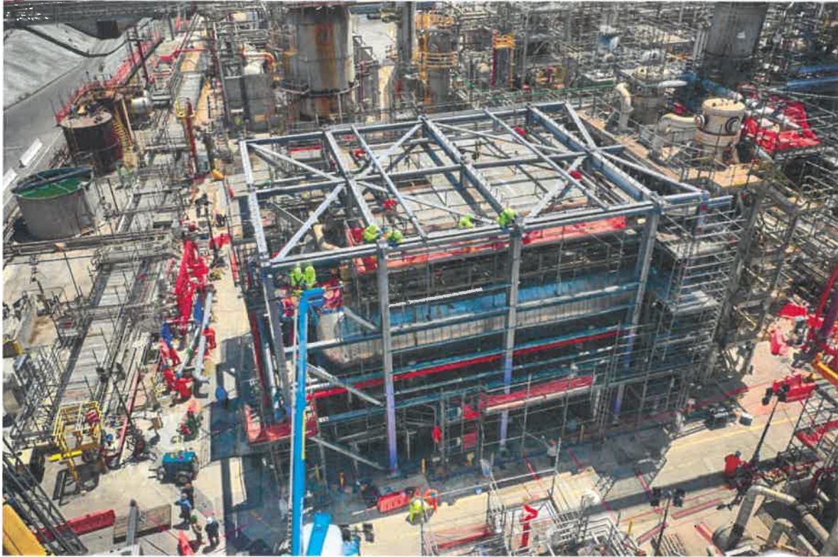
Structure with Roof Panels Set
