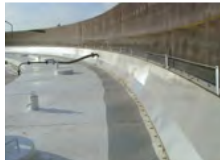
CTS20L secondary seal with direct foam injection.
