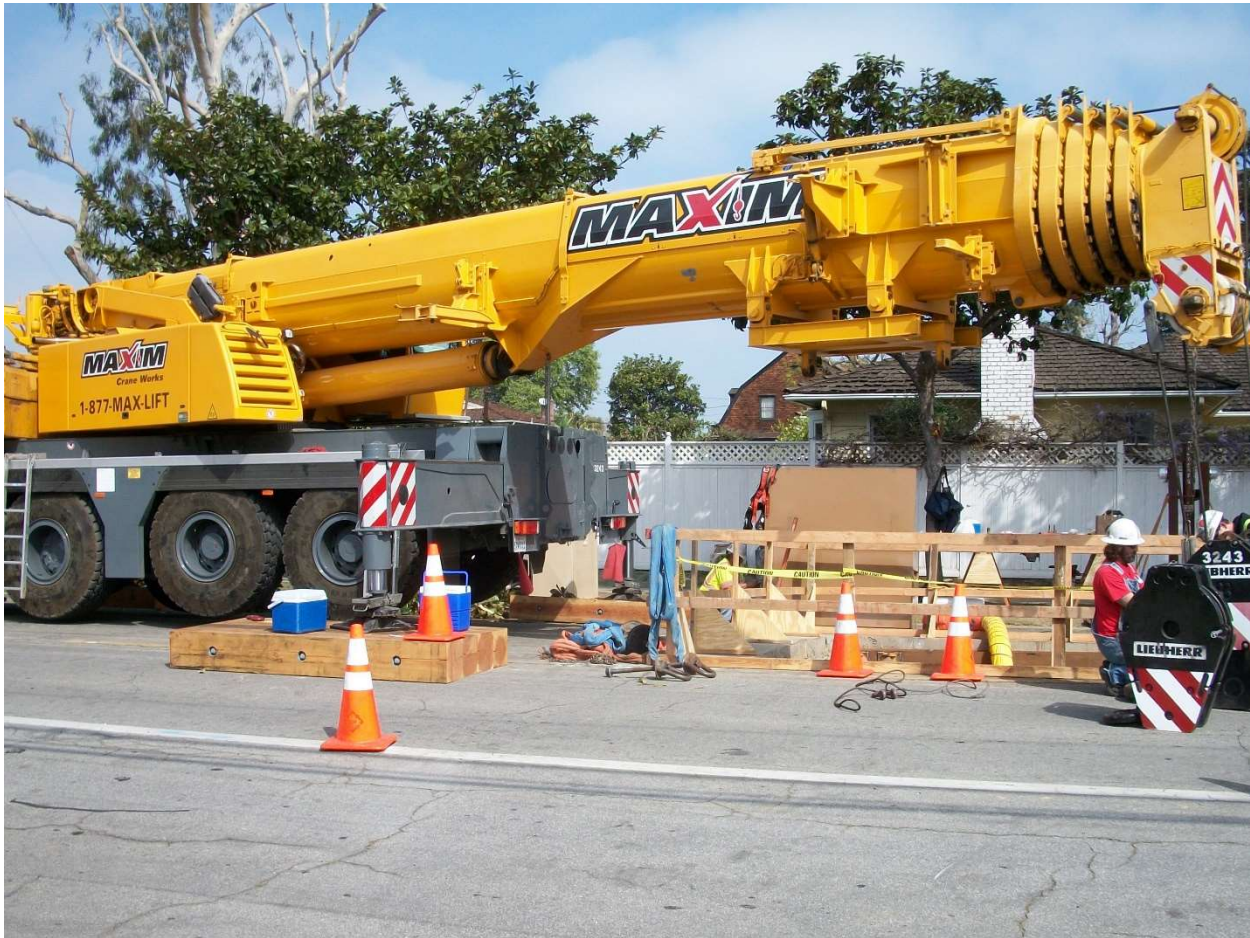
1. Crane lowering a new valve into a trenched section of roadway
