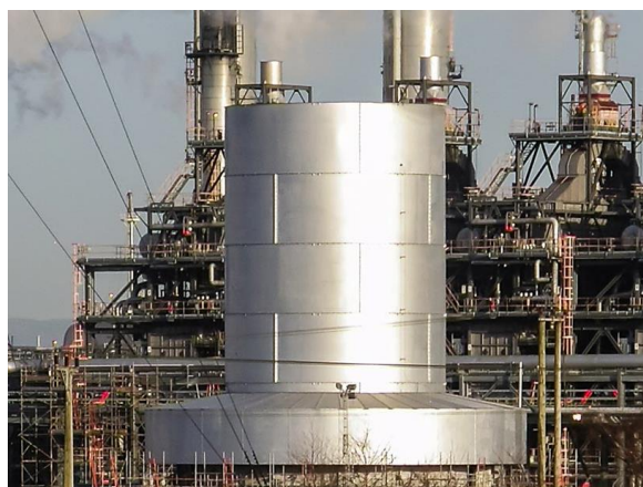
Figure 2-8. Enclosed Ground Flare
