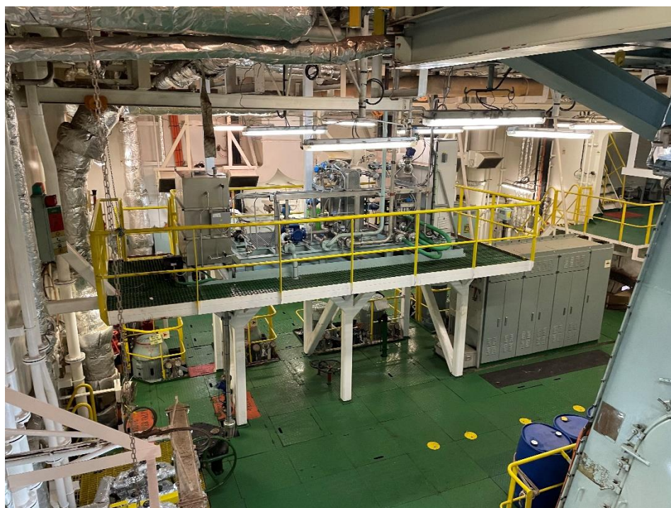
Figure 2 - WIF unit Installation completed
