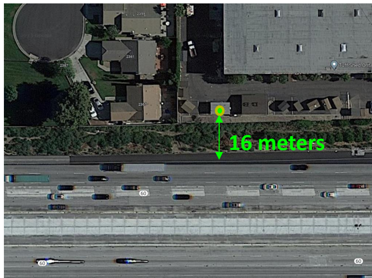
FIGURE 5-10 LOCATION OF THE ONTARIO CA-60 NEAR-ROAD MONITOR
