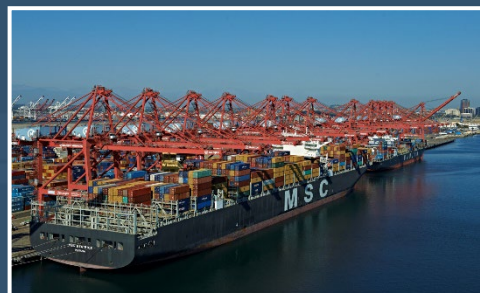
Wilmington, Carson, West Long Beach (WCWLB)
