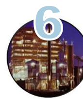
Greenleaf Desert View Power Plant (former Colmac Power Plant)
