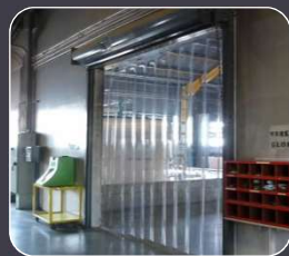
Building Enclosures to Contain Fugitive Emissions
