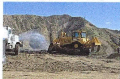
Water Spray While Spreading
