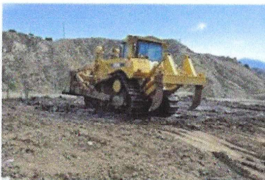
Compacting Wet Debris
