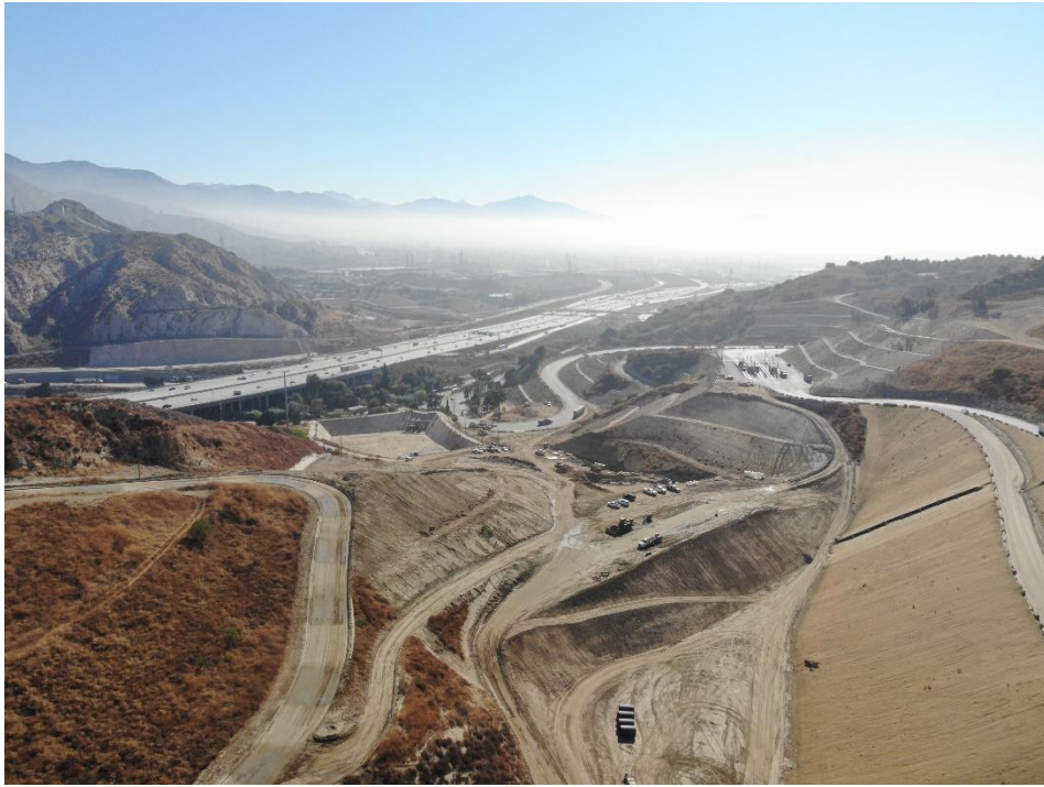
Image 5: View of Toe Berm project, terminal basin and scales.
