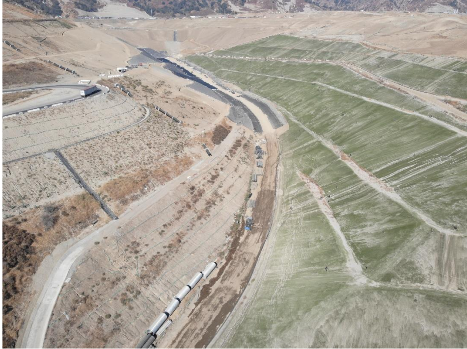
Image 11: View of closure turf and new cell development looking west.
