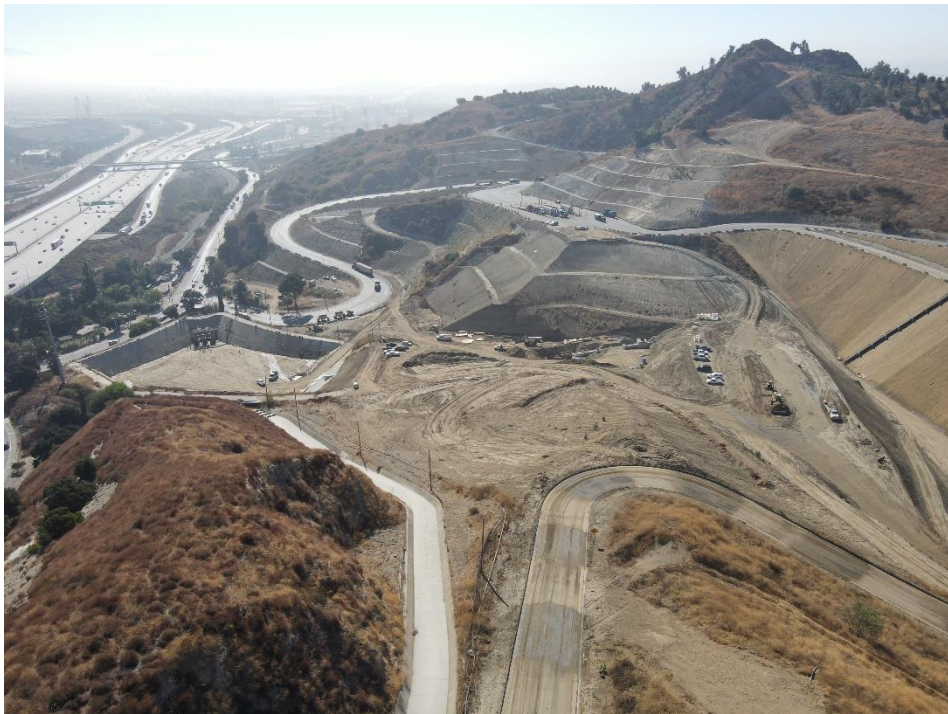
Image 6: View of Toe Berm project, terminal basin and scales.
