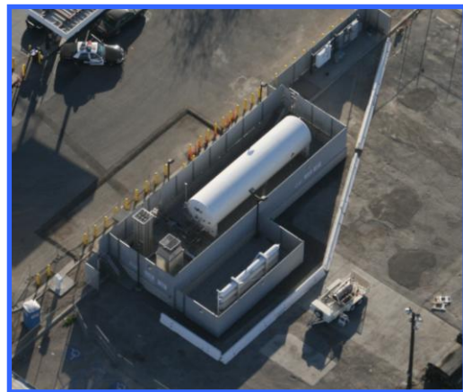
Figure 16: City of San Bernardino’s East Valley Regional Fueling Facility
