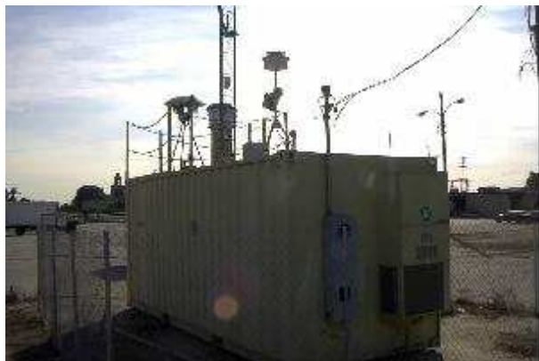
Looking at the probe from the North.
