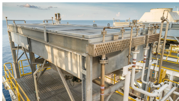
Figure 1-6 - Fin Fan (Source: linkedin.com)
