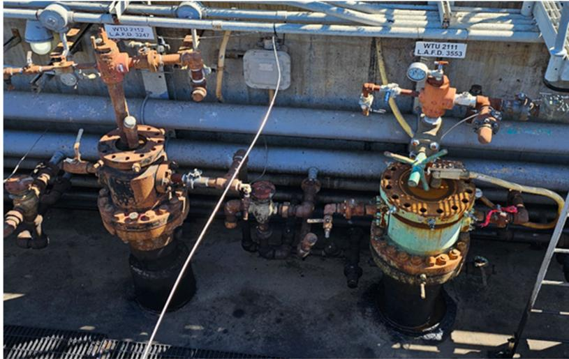
Figure 1.2 – Example of Wellheads Inside a Well Cellar
